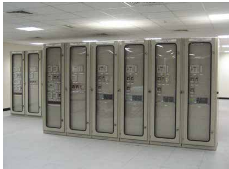
Installation of a substation integrated control system - Bahrain
